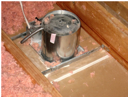
Sealing can lights.
