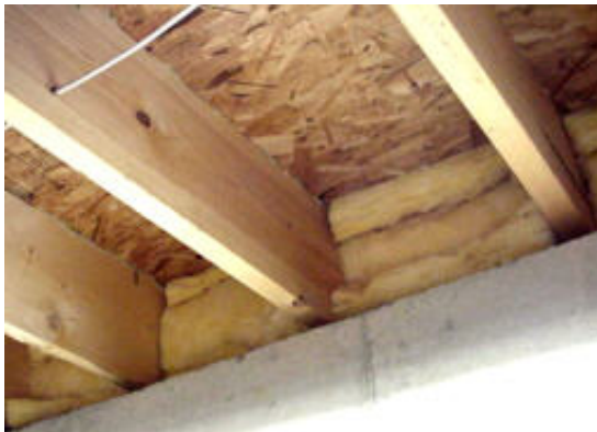
Band joists are a large source of air leakage in the home
