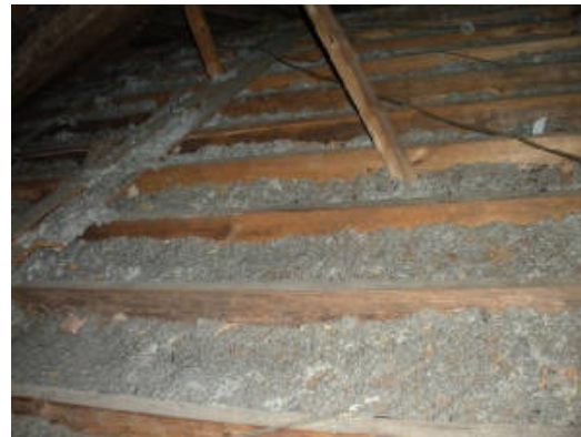
insulation has settled in the sloped ceilings
