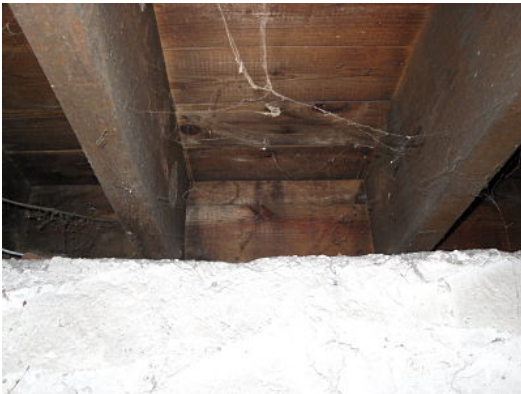
Band joist insulation can be upgraded once air-sealed
