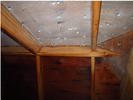
frosting on roofing nails indicates elevated attic moisture
