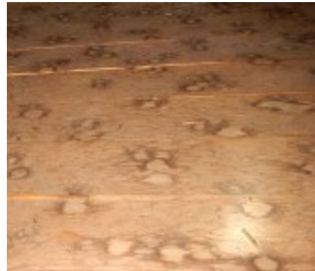
drip from roof, no perceivable leak, presumed condensation
