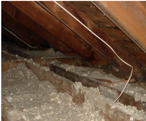
Room exists to add more insulation after air-sealing
